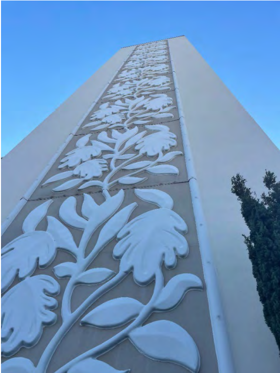
Figure 53A. Fiberglass decorative plates on front face
