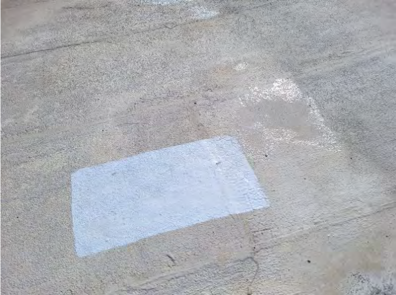
Figure 41 Previous repair made to roof
