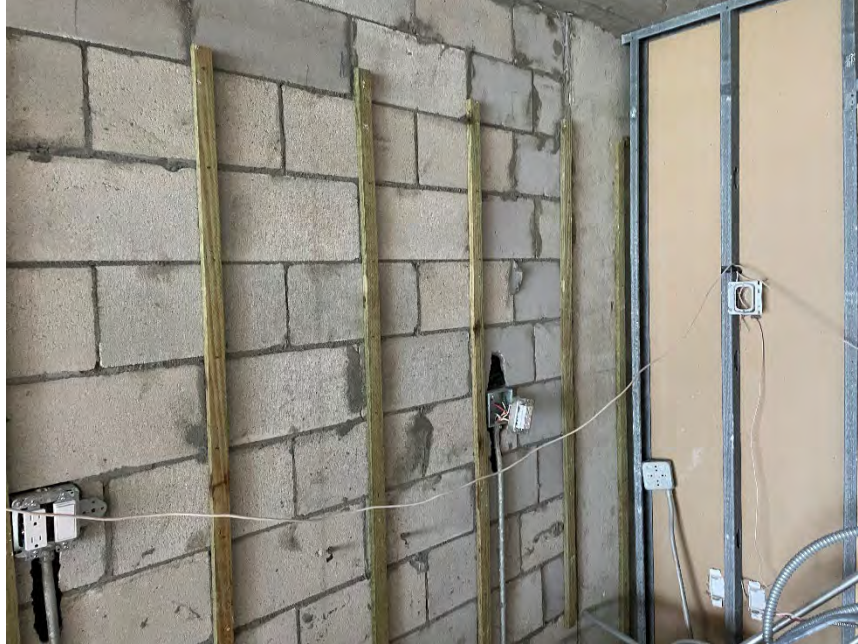
Figure 7 Typical Dividing CMU wall and metal framed wall in Unit 606
