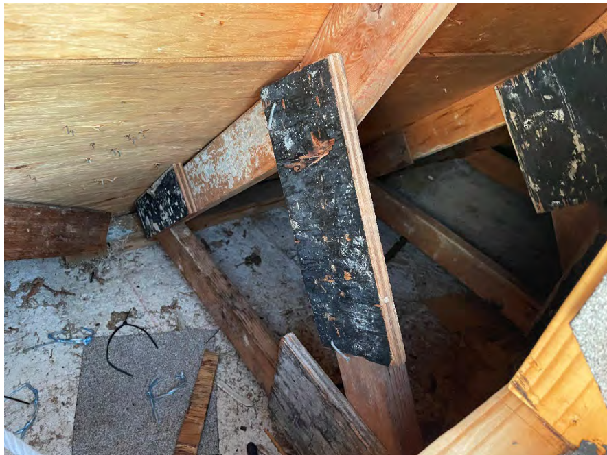
Figure 47 Access hatch confirming construction atop modified bitumen roofing
