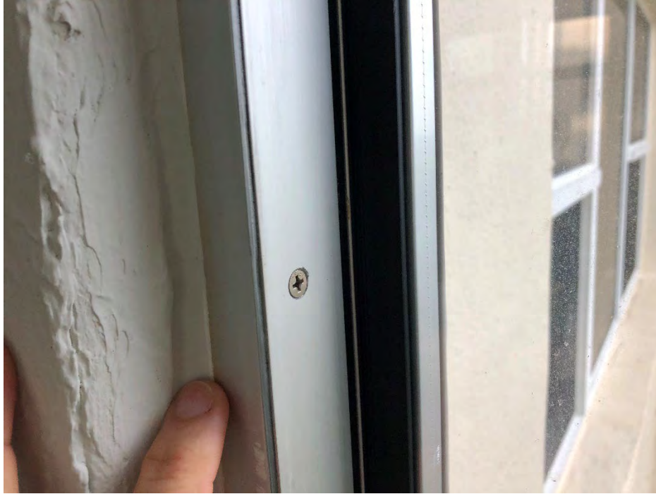
Figure 59 Interior Sealant at Lanai windows
