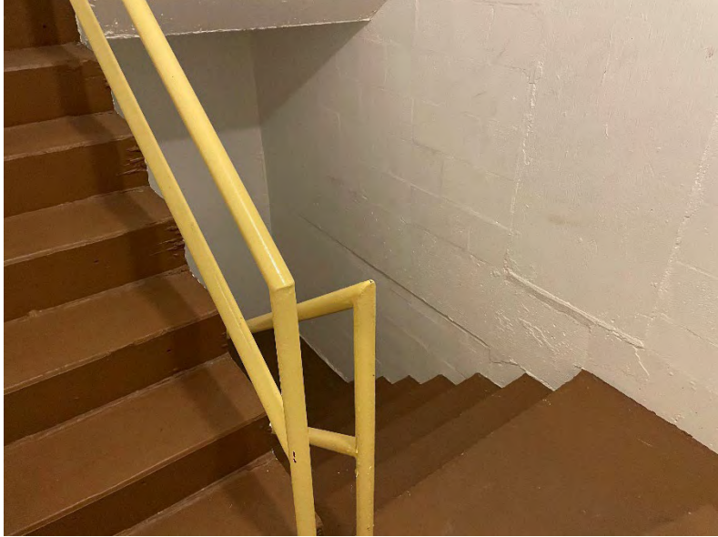
Figure 5 CMU construction in the stairwells
