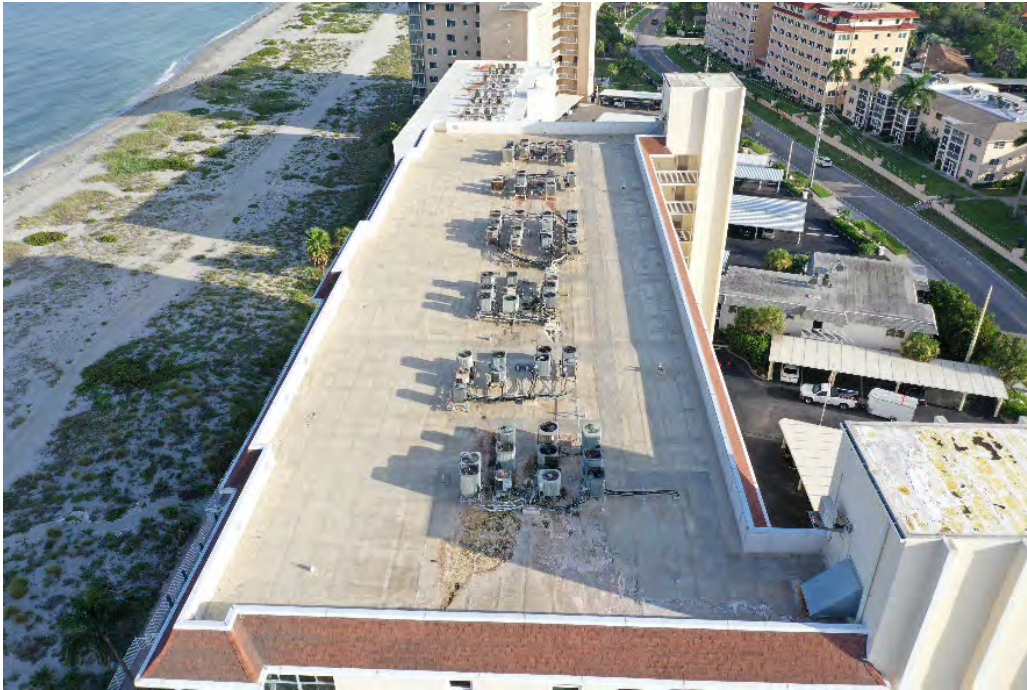
Figure 31 Roof at Gulf Shores with a recoat applied
