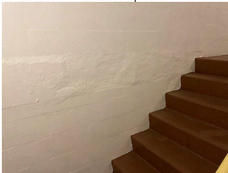
Figure 18 Floor terminating in staircase
