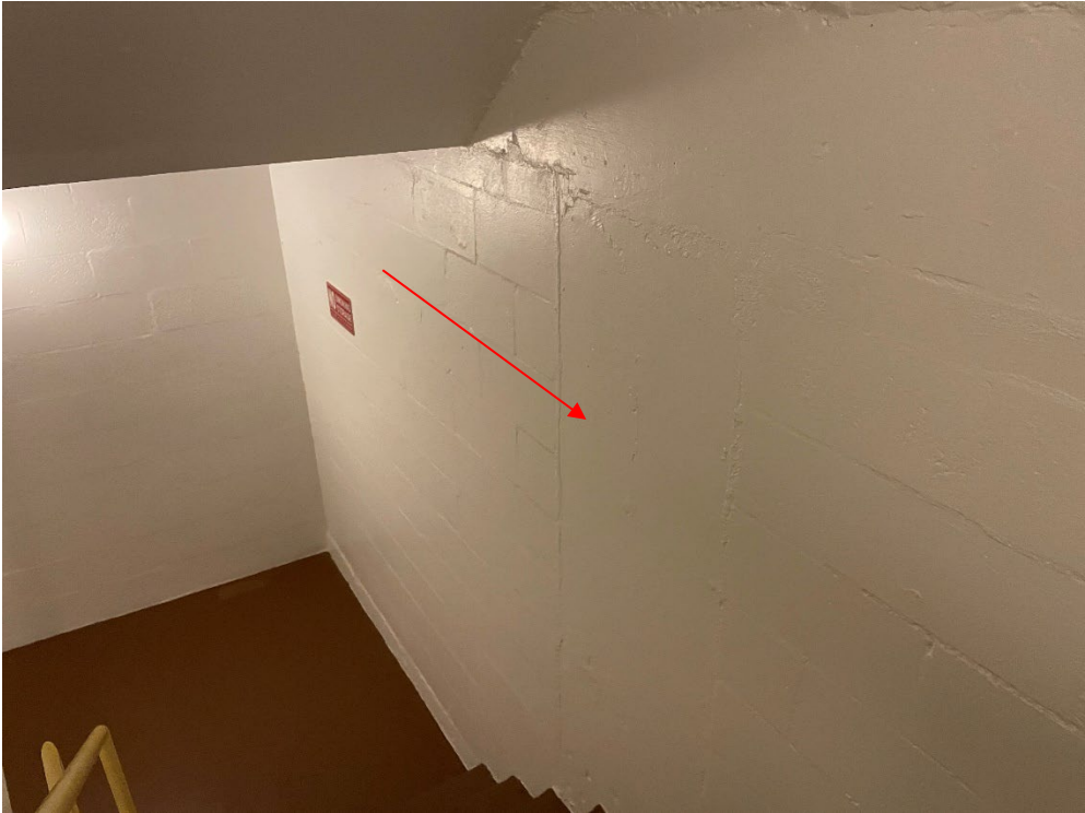
Figure 13 Stairwell ties into columns
