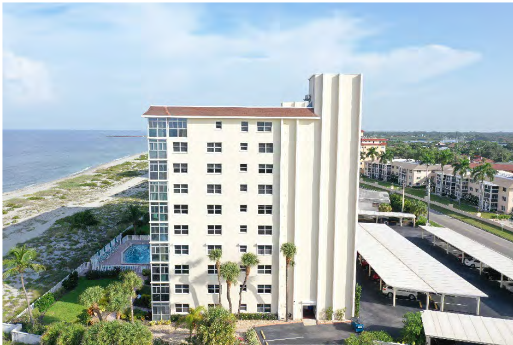
Figure 48. General View of Stucco and Paint
