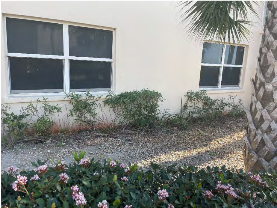
Figure 52. Plants close to exterior of building on north side
