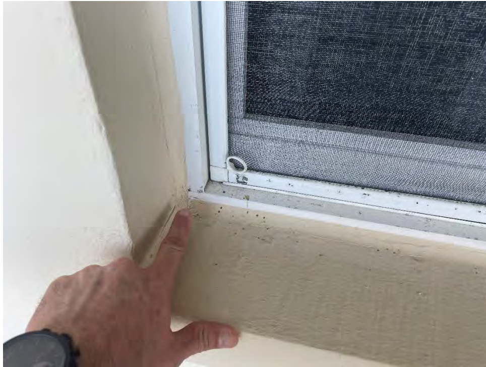
Figure 56 Exterior Sealants appear adequate on walkways.
